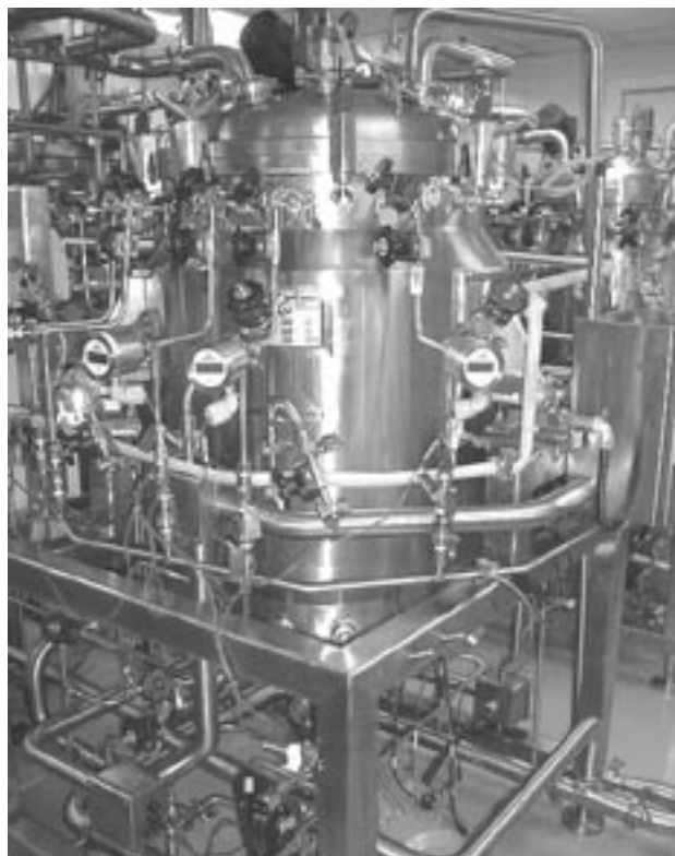
Fermentation Facility at NCP's Headquarters
